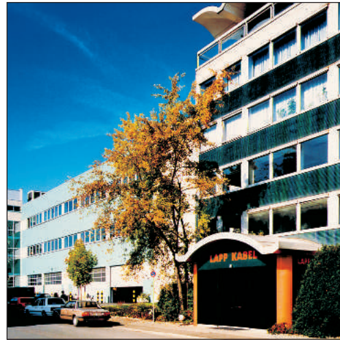
The Lapp Kabel headquarter in Stuttgart-Vaihingen.
